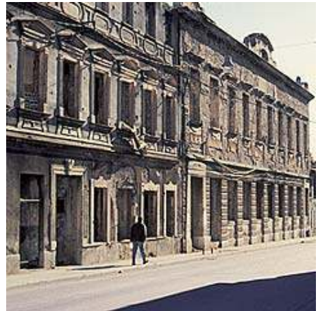
The Pavarotti Music Centre before rebuilding, standing amidst the ruins that continues today to be East Mostar
